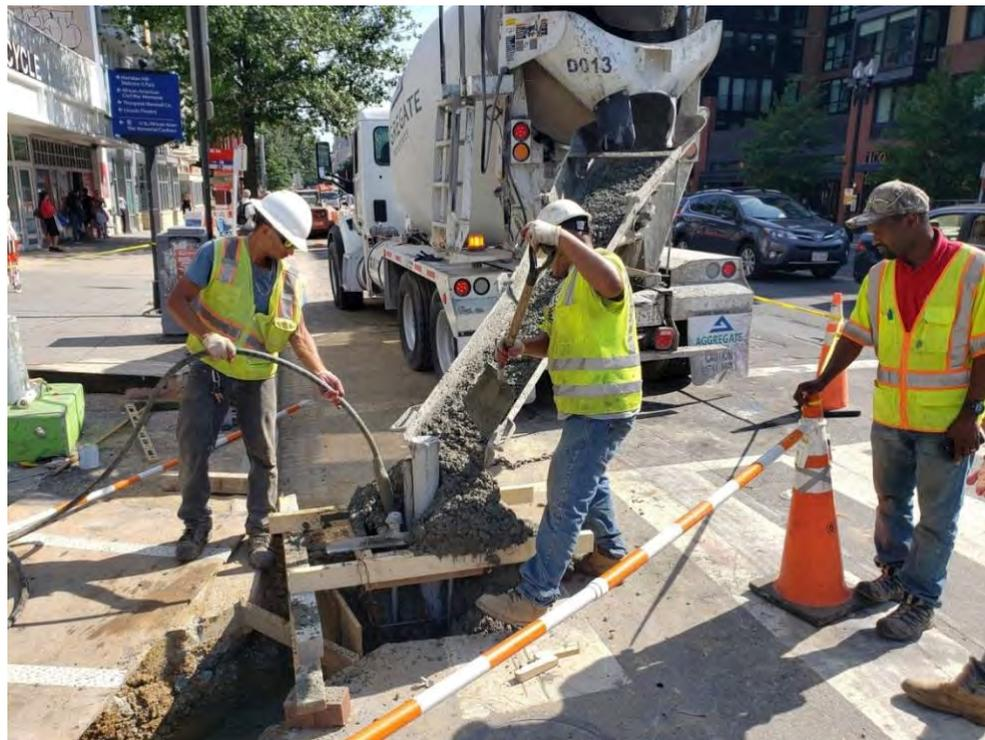
OMNI Pouring traffic pole foundation at 14<sup>th</sup> St. NW & U St.
