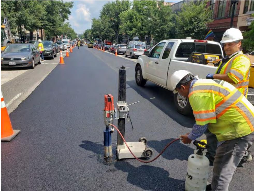
Geo-Tech Subcontractors collecting asphalt samples for testing
