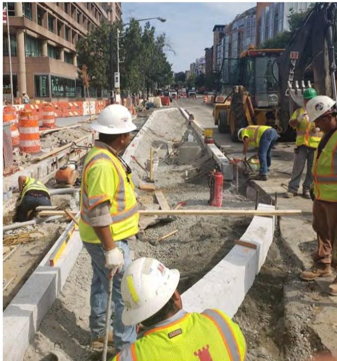
Bus Island granite curb installation at 14<sup>th</sup> St. NW & U St.
