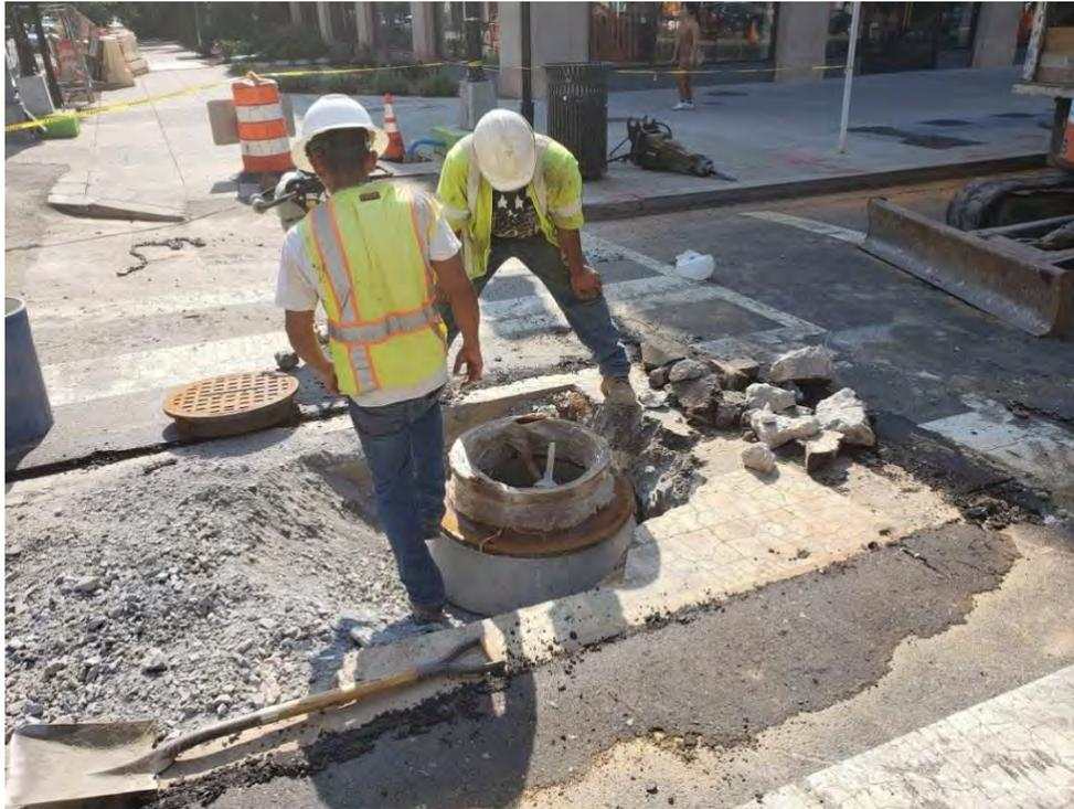
Adjusting manhole elevation to match finish grade at 14<sup>th</sup> St. & R St. NW
