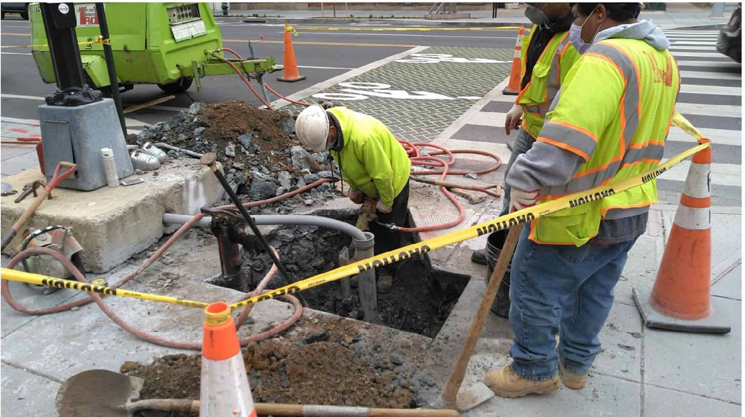
FMCC Restoring damaged Signal foundation at Q street
