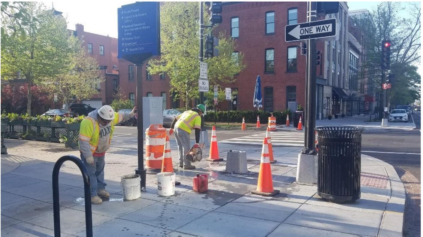
FMCC working on removing the T-base at NEC of Q Street
