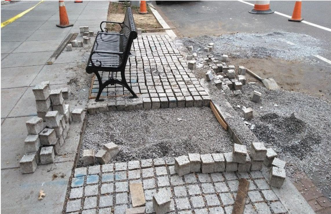
DEN installed geo grid and reinstalled in half of this location in front of the Studio Theater on NB 14<sup>th</sup> Street NW
