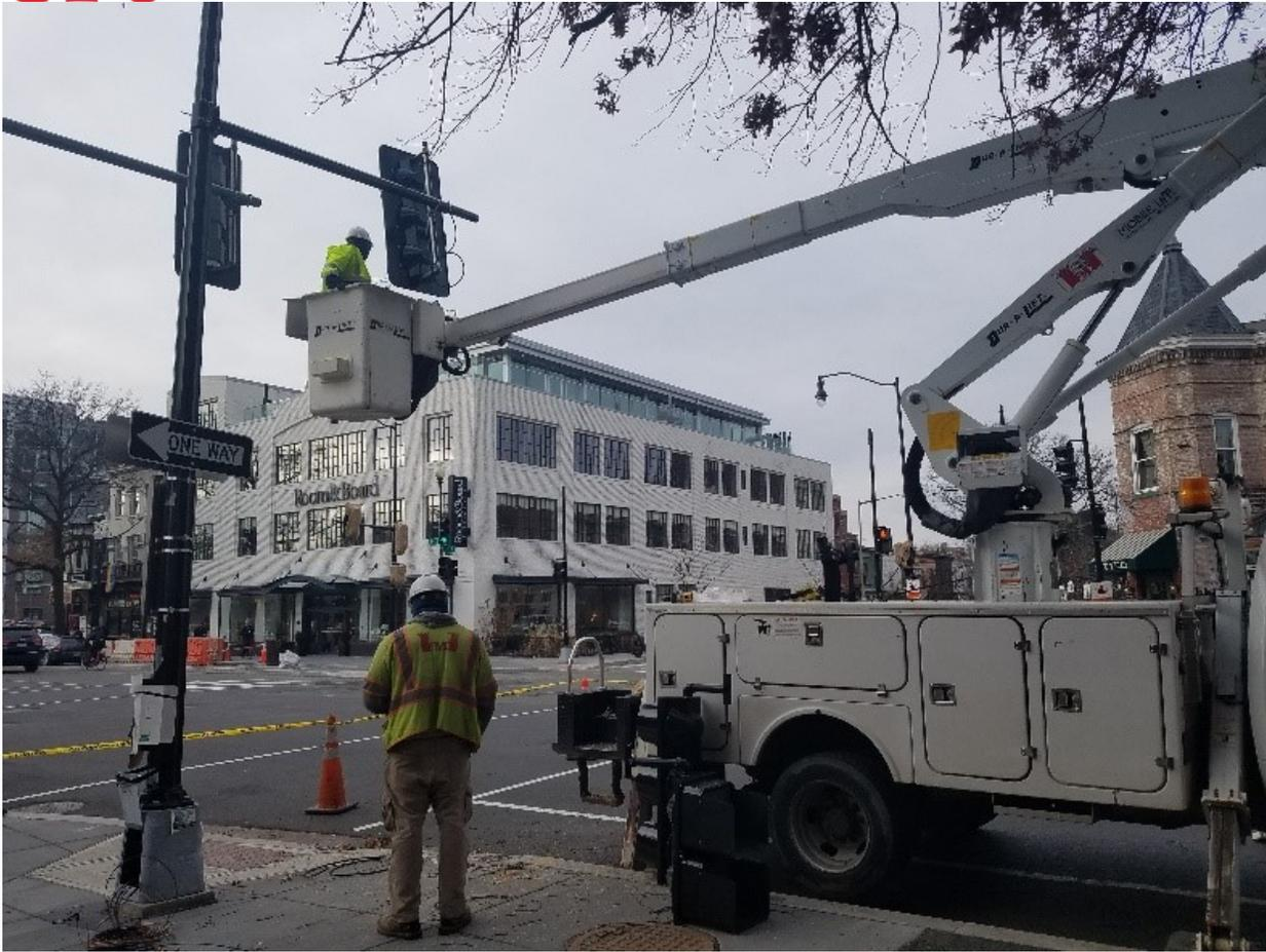
Mast arm and 3 section installed at L-87
