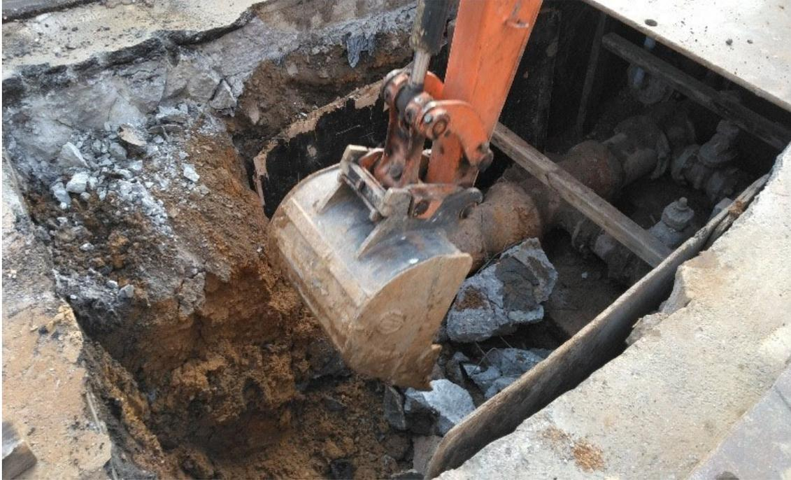
Omni enlarging the hole for the water main tie in at SB 14<sup>th</sup> Street NW at R Street
