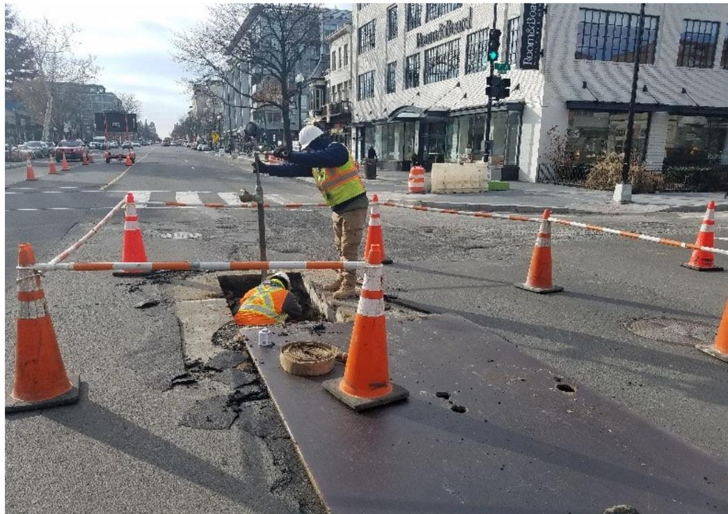
Omni Excavators preparing for water main pressure test between T and Wallach St
