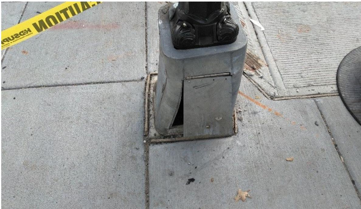
The damage to the light pole base and foundation from the accident at NW corner of Q Street & 14th Street NW
