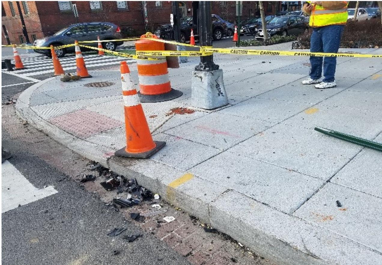
Traffic signal foundation, base and pole TS-21 damaged by car at NWC of 14<sup>th</sup> & Q St
