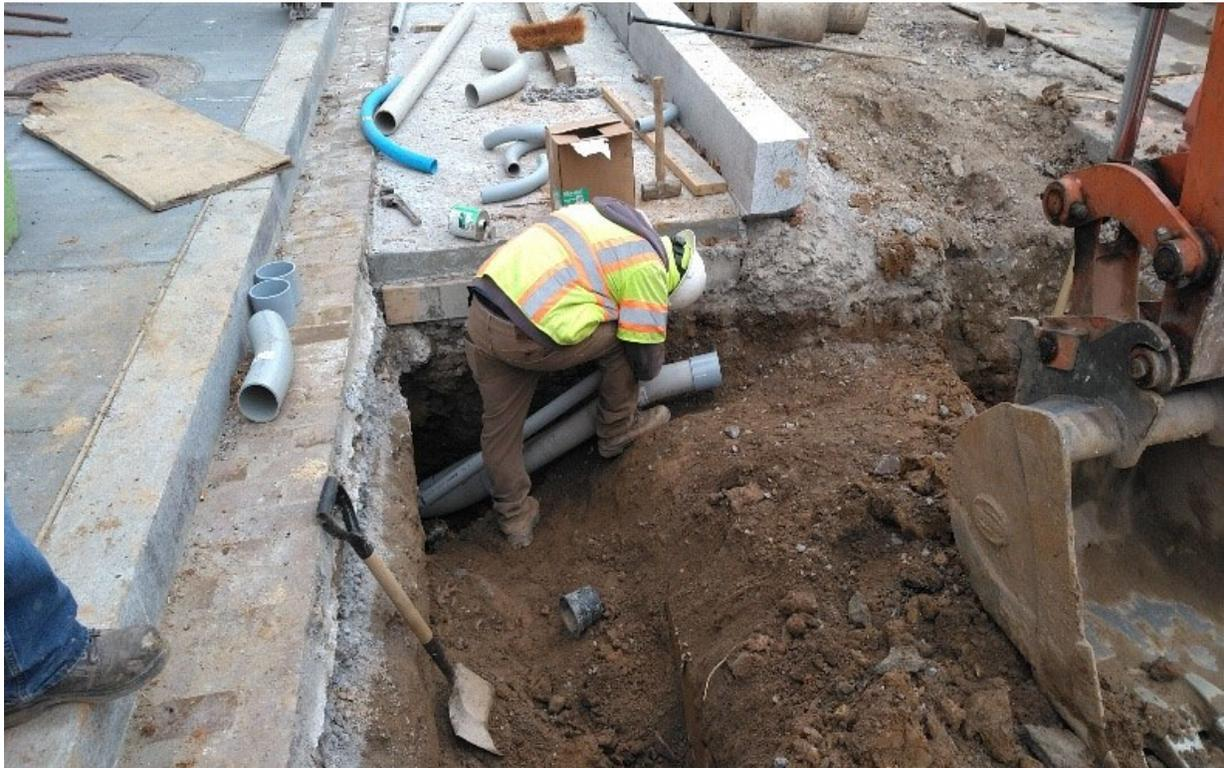
Omni installing 2 EA 2" & one 4" PVC conduits for the Bus Stop Nand box and pedestrian signal at SB 14<sup>th</sup> Street & R Street
