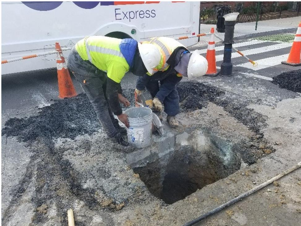
Excavation of roadway for missing water valve at NWC of 14<sup>th</sup> & Q St by Omni
