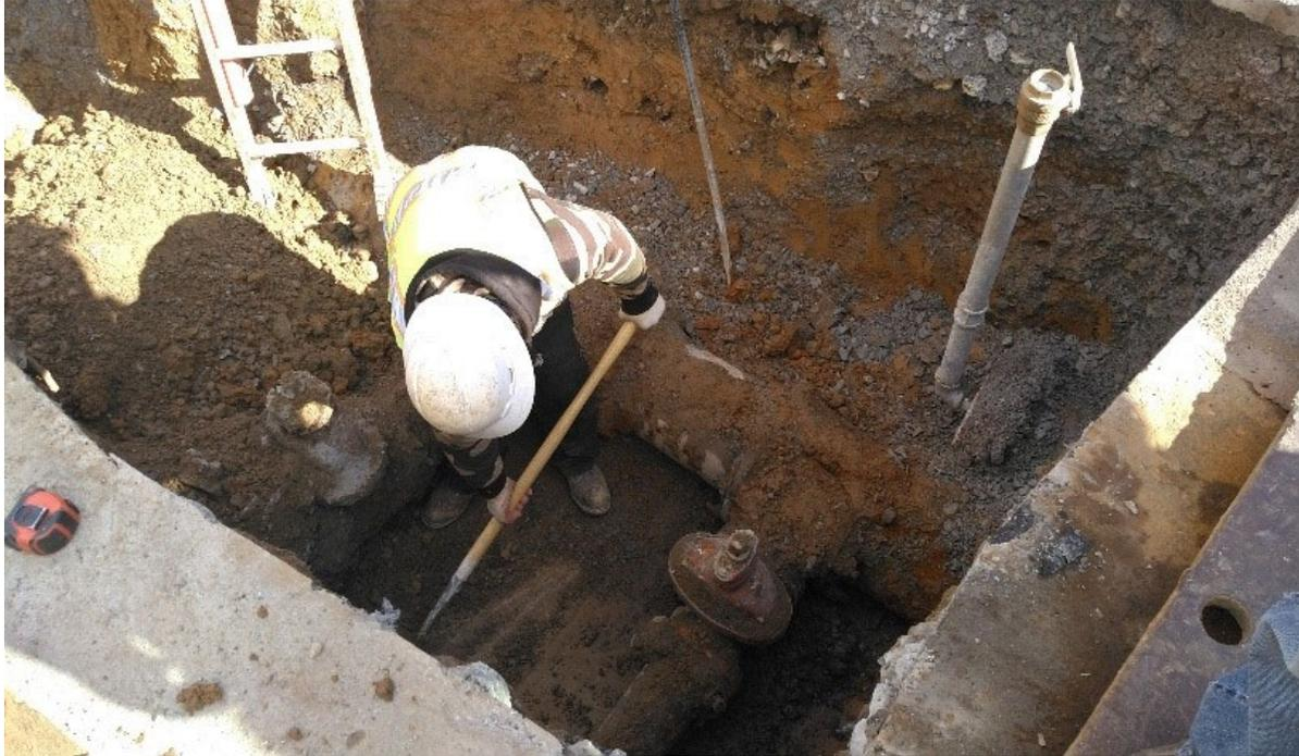
Omni continuing to hand dig around the water mains at 1SB 4<sup>th</sup> Street NW at R Street
