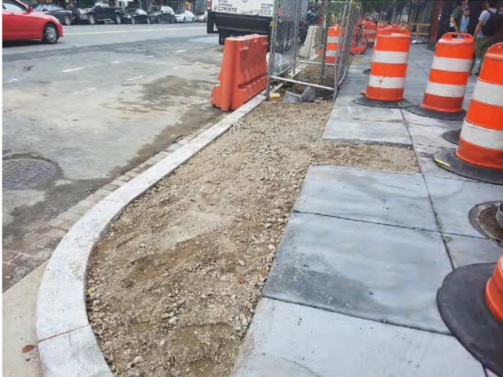
*Backfilling Tree Space area to remove MOT between N Street and Rhode Island*
