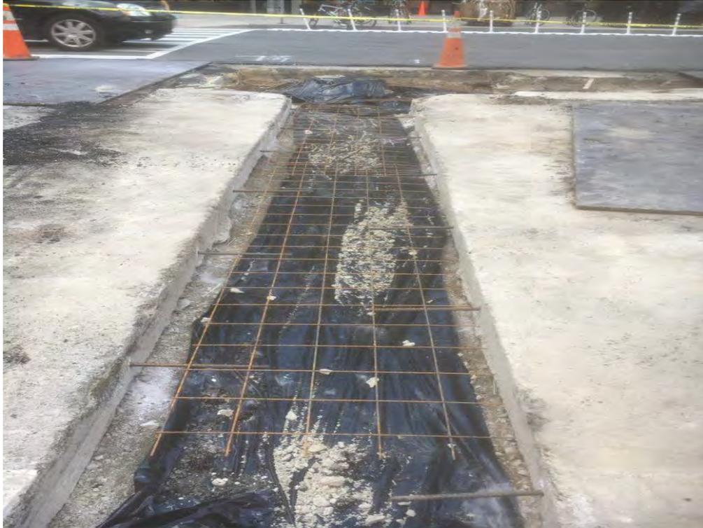
*Wire mesh and Rebar prior to placement of PCC Base on Wallach St.*
