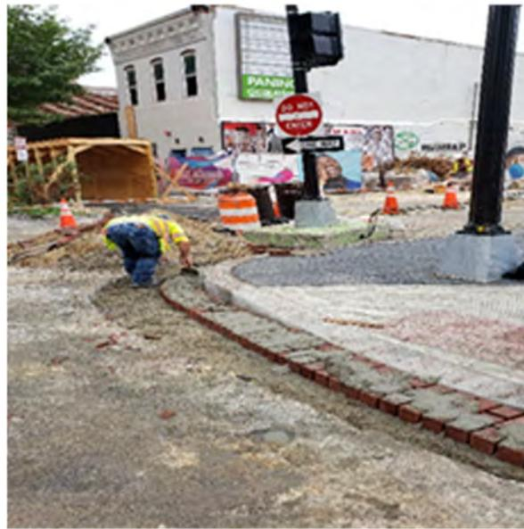
D.E.N. crew also installed and placed 63.4 LF of Brick Gutter at 14<sup>th</sup> St. & W St. Crosswalk area.
