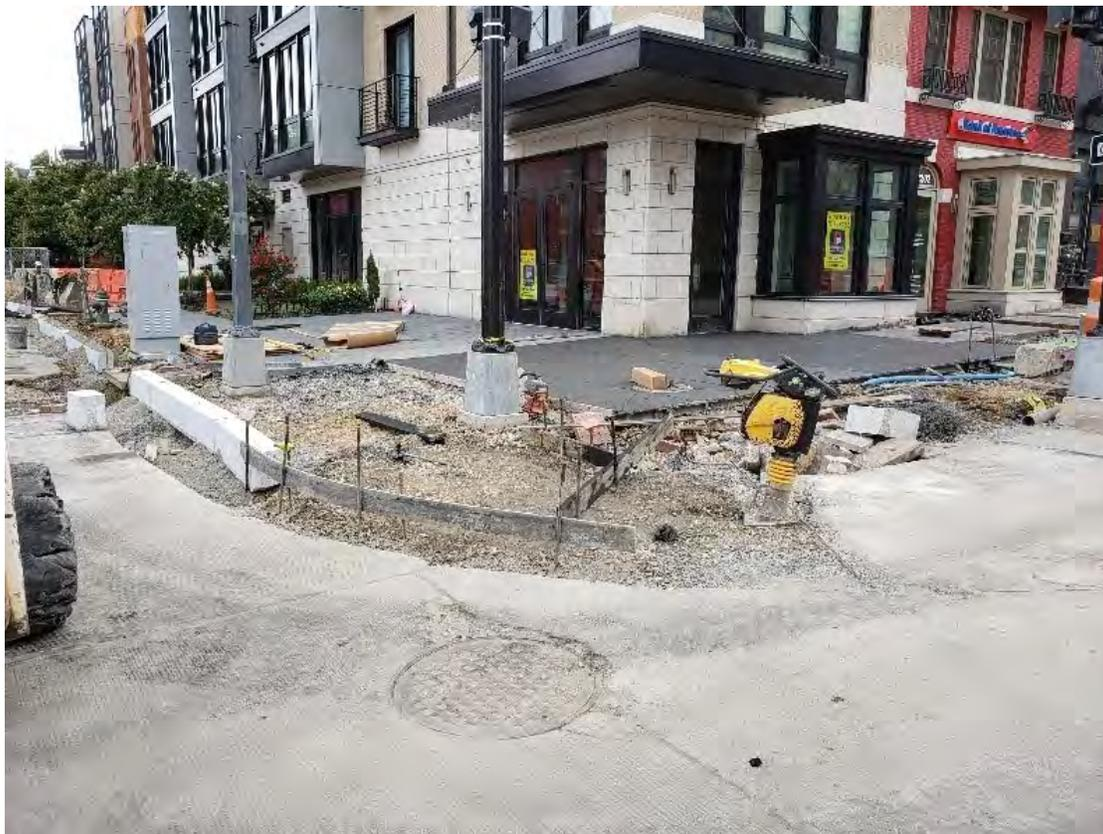
D.E.N crew demoed & Removed Ex. Curb and Gutter, Old Ramp and adjusted 2 Utility Manholes prior to placement of Class F Concrete.
