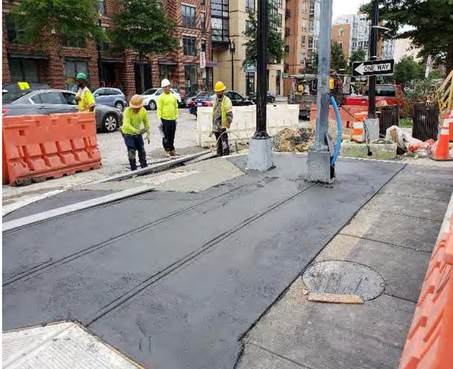
DEN crew adjusted 2 Utility Manholes at the Sidewalk at NWC of 14<sup>th</sup> ST. & W St. NW.
