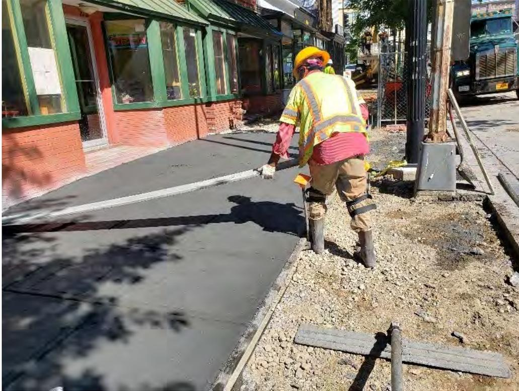
D.E.N placed and finished Concrete sidewalk from 2208 thru 2212 Blocks of 14<sup>th</sup> St. NW at SB.
