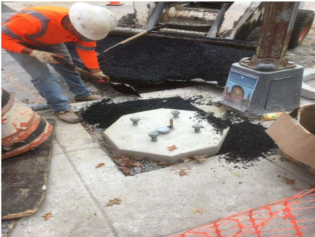
*Placement of Temporary Asphalt around previously poured Street Light Foundation*
