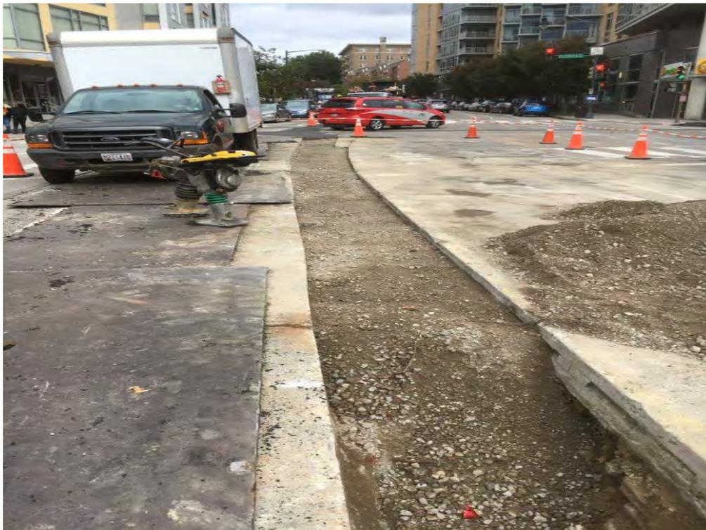
*Backfill of Encased Electrical Trench between Florida and W Street*
