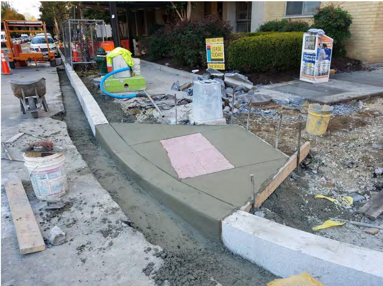
*Installation of ADA Ramp at the NW corner of 14<sup>th</sup> and N Street on the N Street side*
