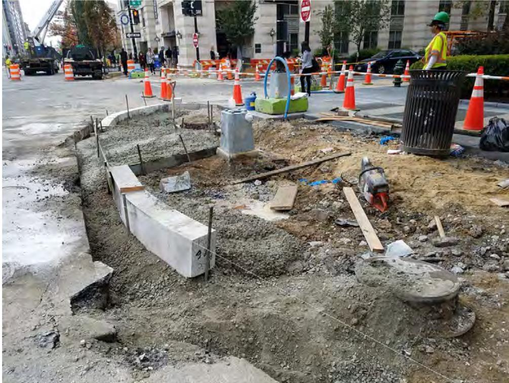
*Installation of Granite Curb for Bulb Out at NW Corner of N Street*
