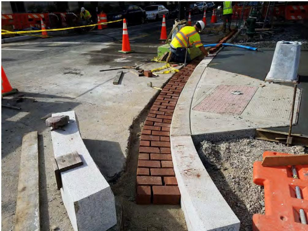
*Placing Brick Gutter at the NW Corner of 14<sup>th</sup> and N Street*
