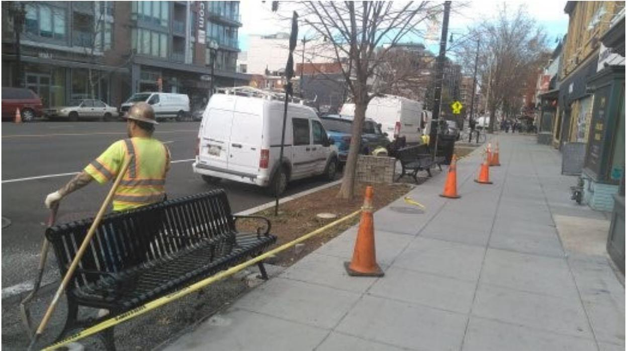
DEN removing the permeable pavers to install geo grid at 1805 14<sup>th</sup> Street NW
