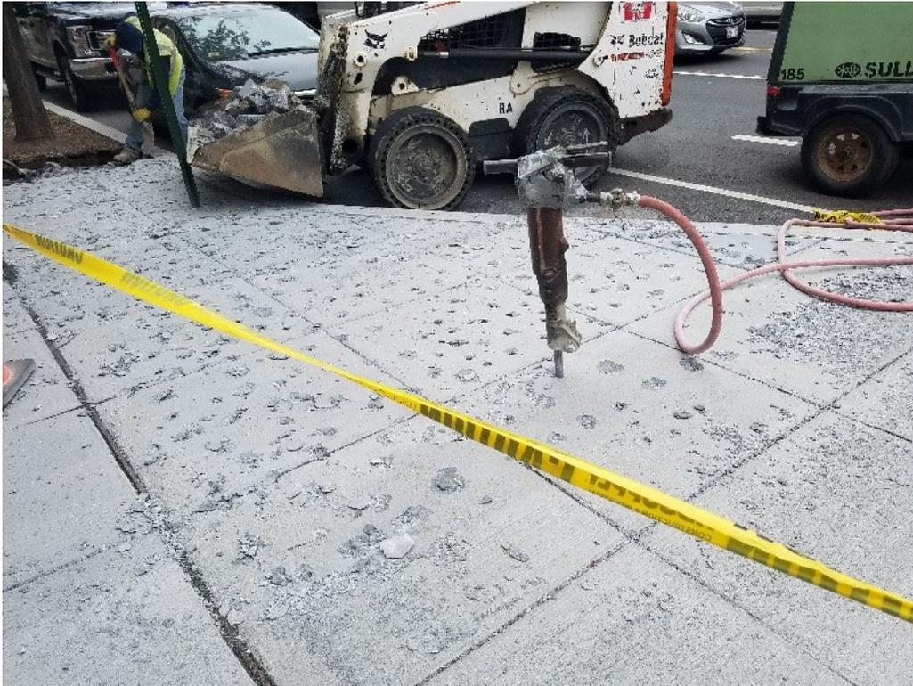
D.E.N. demolished SEC of 14<sup>th</sup> & Q St PCC sidewalk for tree planter area.
