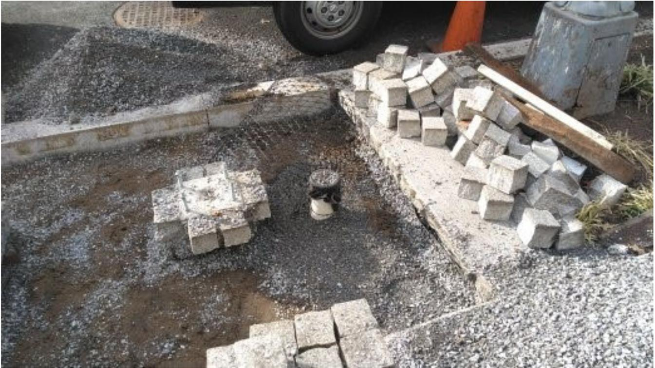
DEN removed the permeable pavers at 1807 14<sup>th</sup> Street NW to install the geo grid and a observation well
