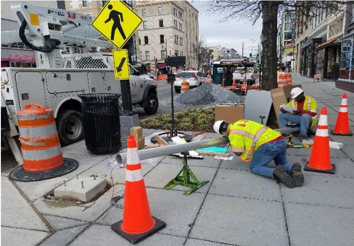
FMCC electrical crew at NEC of 14<sup>th</sup> & Corcoran St installing flashing beacon system
