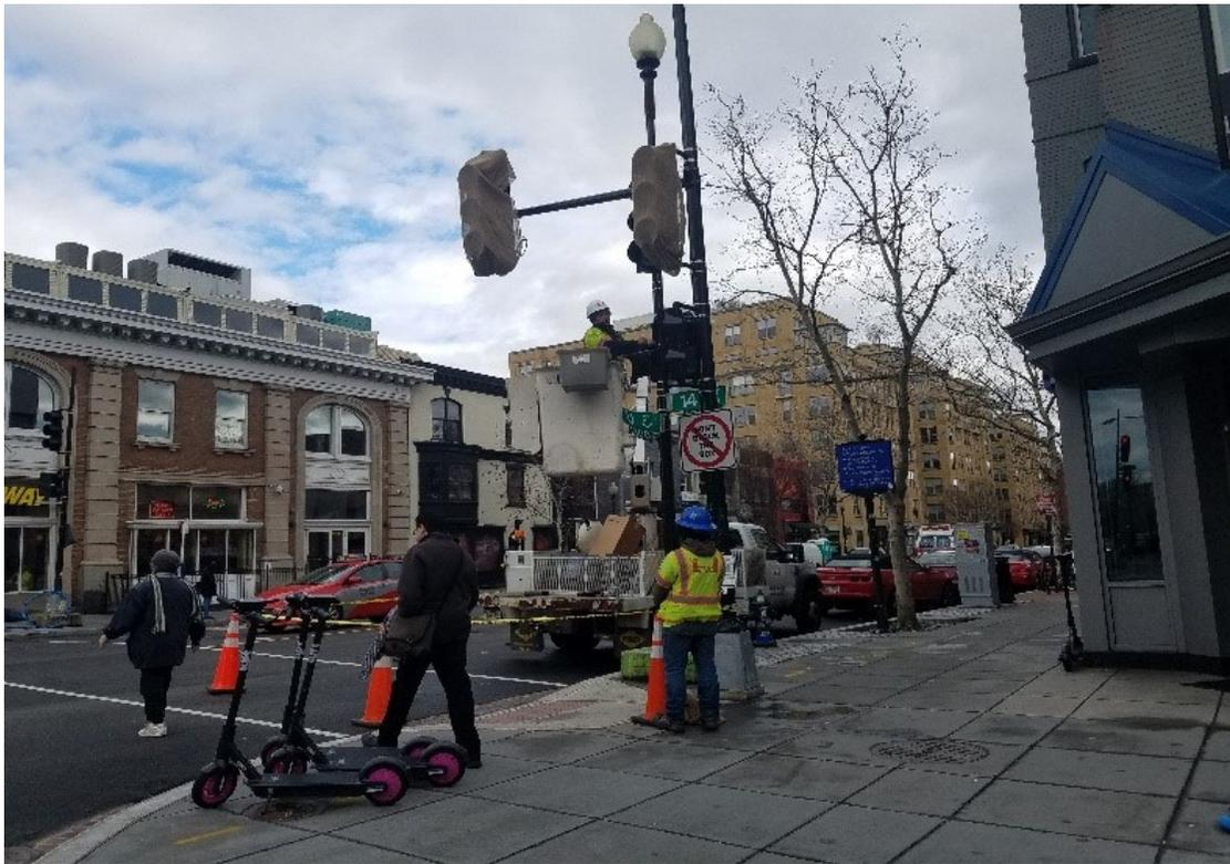
FMCC electrical crew at SEC of 14<sup>th</sup> & Corcoran St installing flashing beacon system
