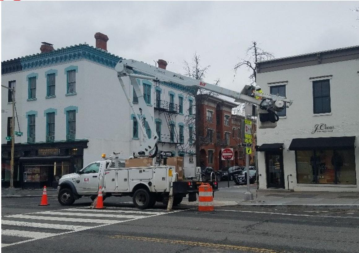
FMCC electrical crew at NWC of 14<sup>th</sup> & Corcoran St installing flashing beacon system
