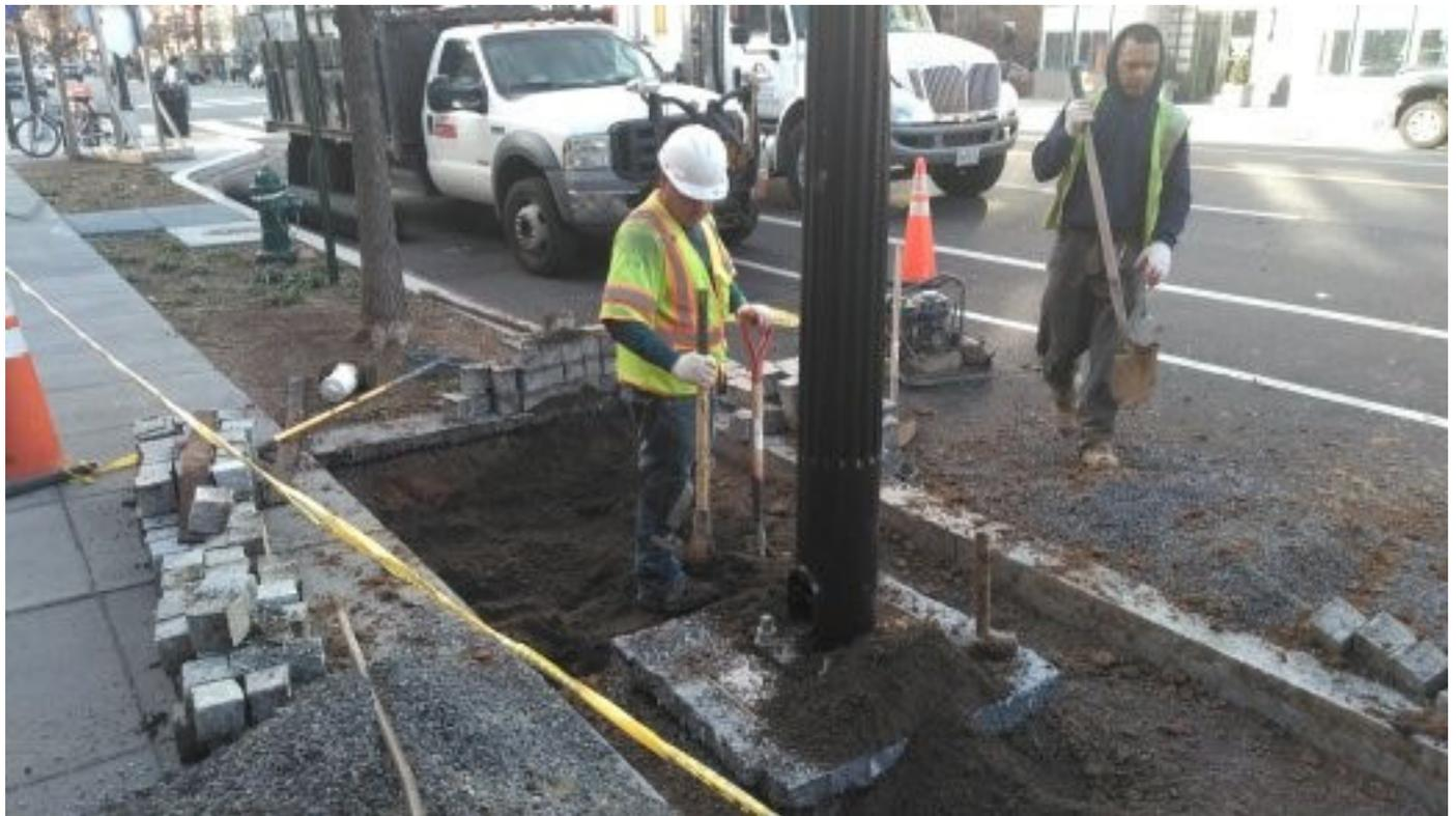
DEN excavating for structural soil prior to reinstalling the permeable pavers at NB 14<sup>th</sup> Street across from the LA Diplomat Restaurant
