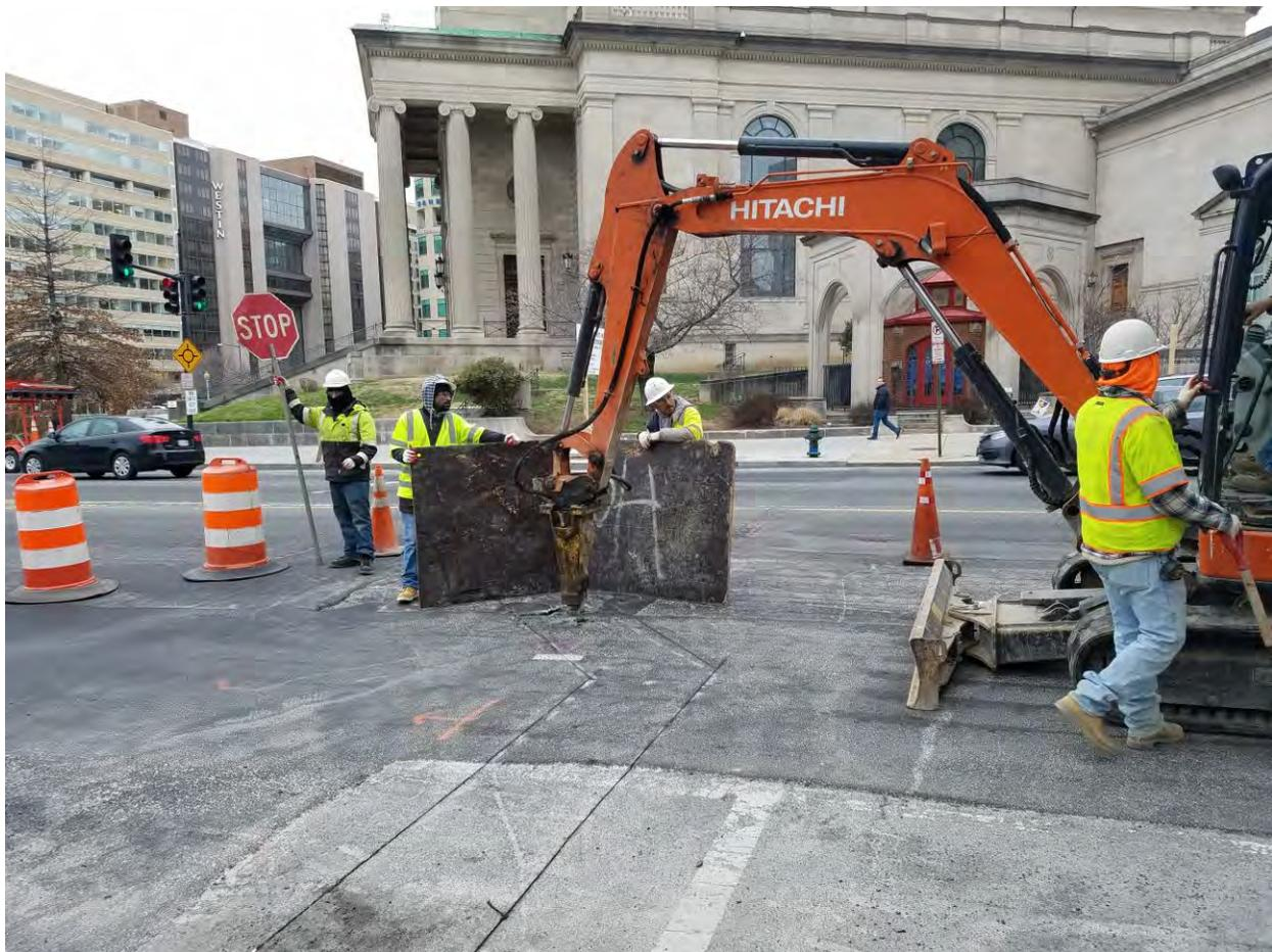
*Demolition of pavement for conduit installation between Thomas Circle and N Street on the Eastside*
