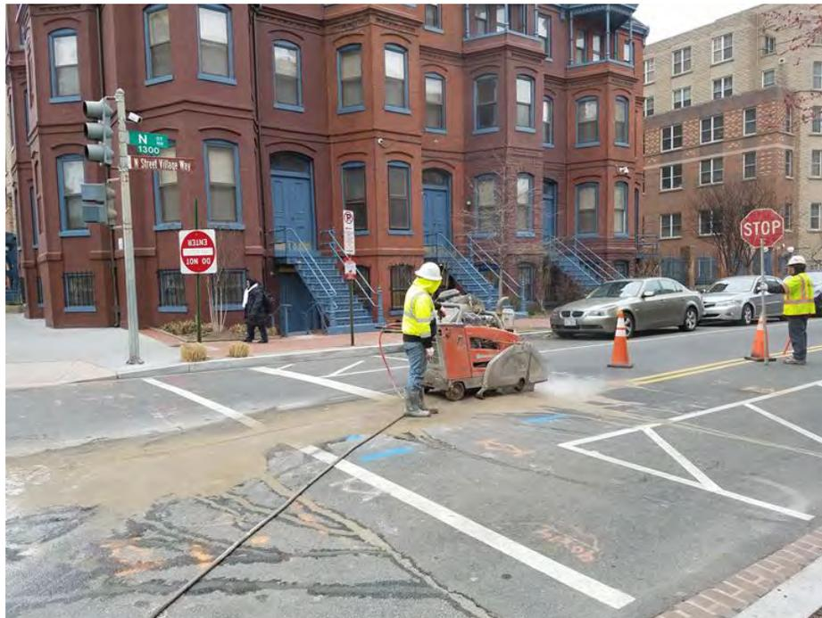
*Saw-Cutting on N Street for Manhole installation*
