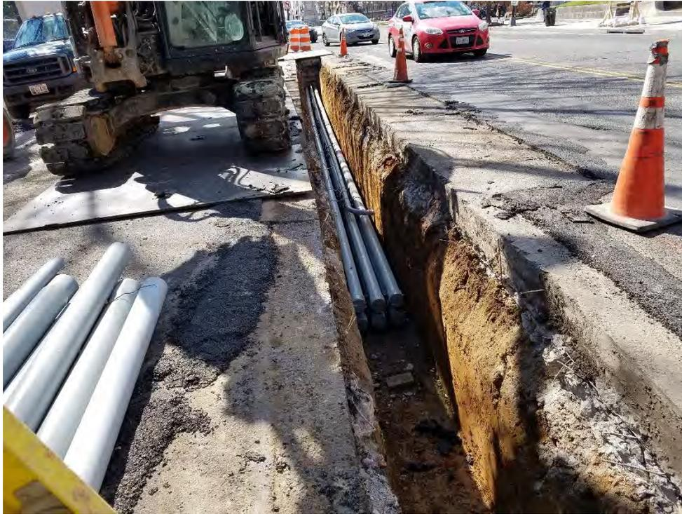
*Installation of 6-4" and 1-2" PVC Conduit*
