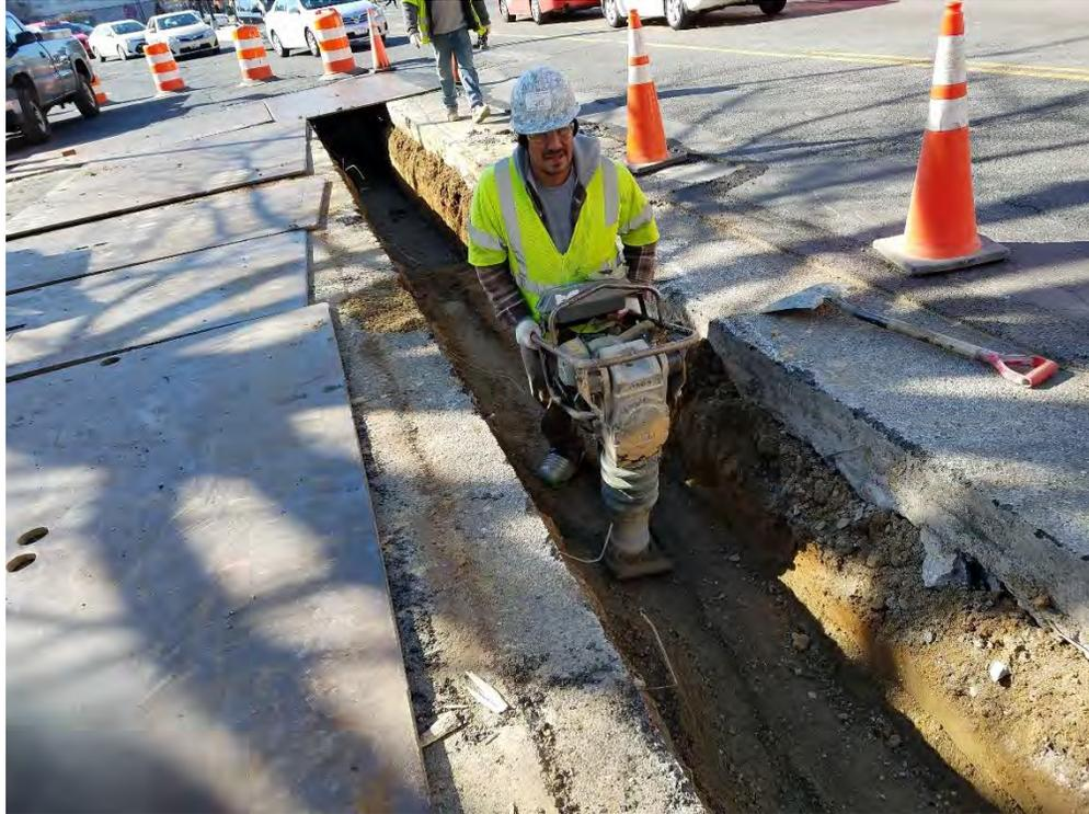
*Compaction of Backfill Material over encased PVC Conduit*
