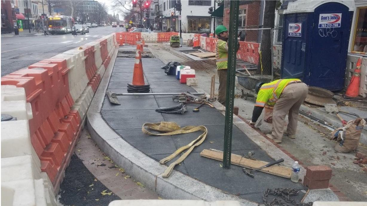
Finished installing brick gutters at the bus island at NWC of T Street
