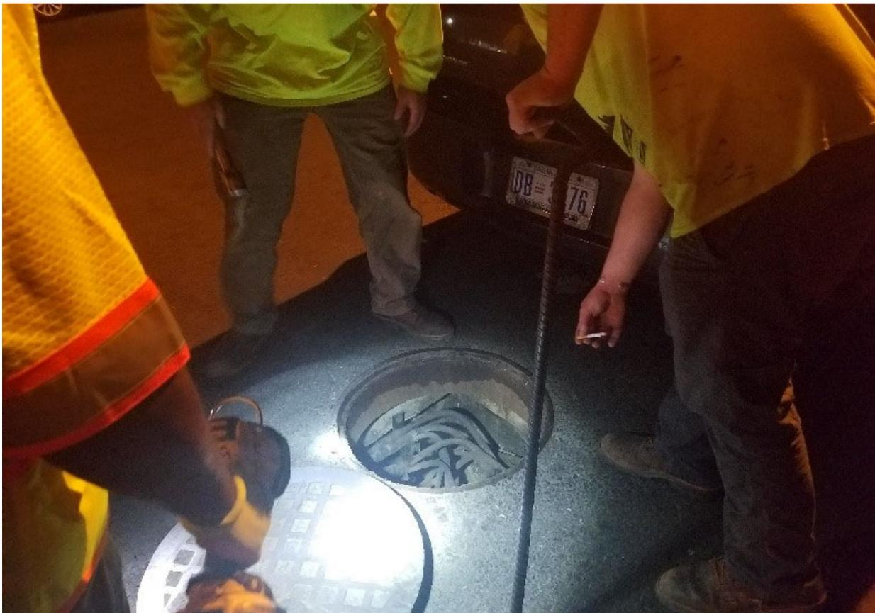
Pepco manhole with communication cable to be removed and replaced.
