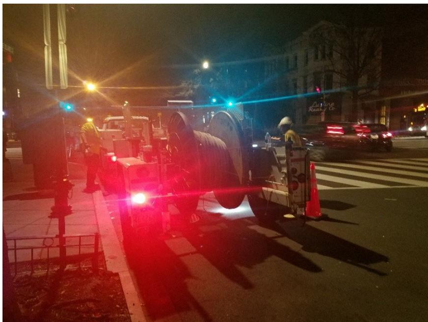
Spool truck to be used to run new cable to Pepco manhole.
