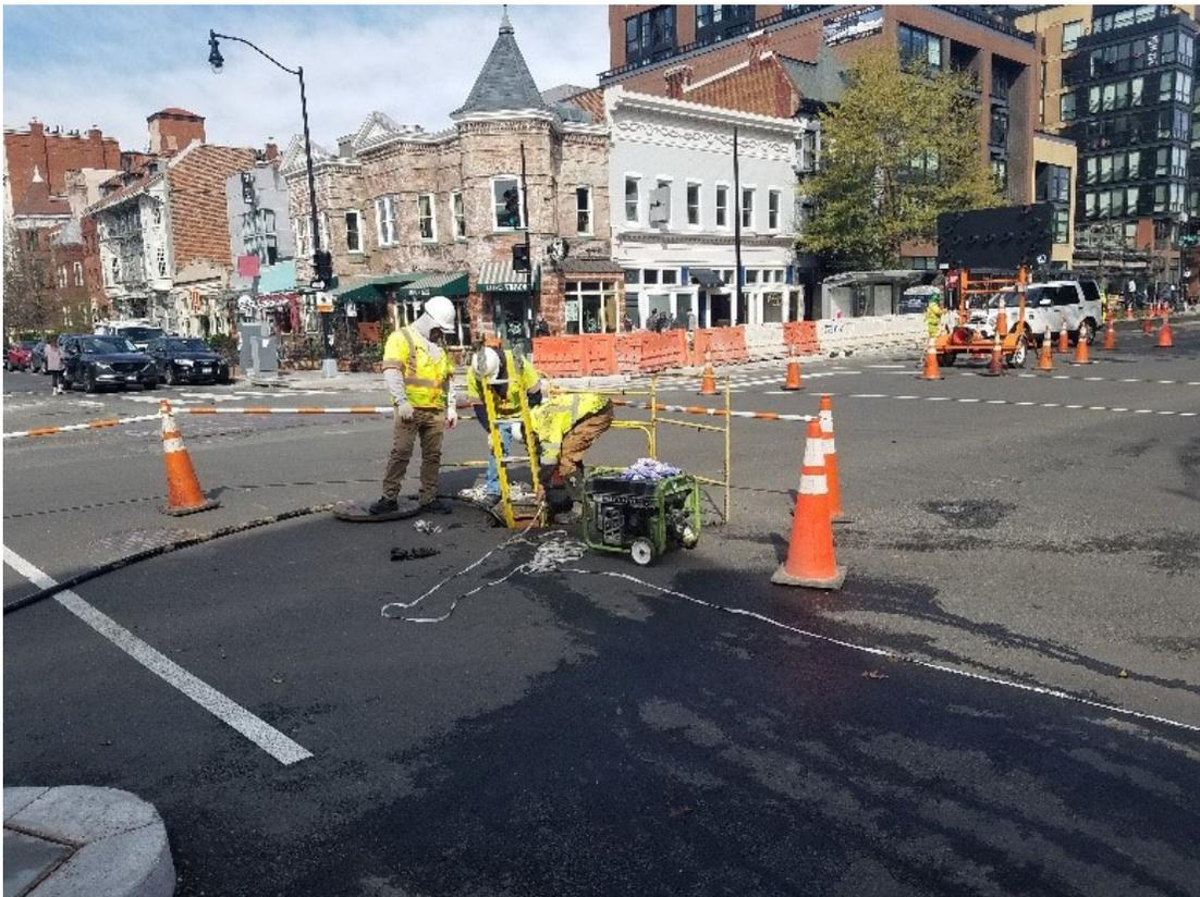
FMCC splicing cable at manhole M66
