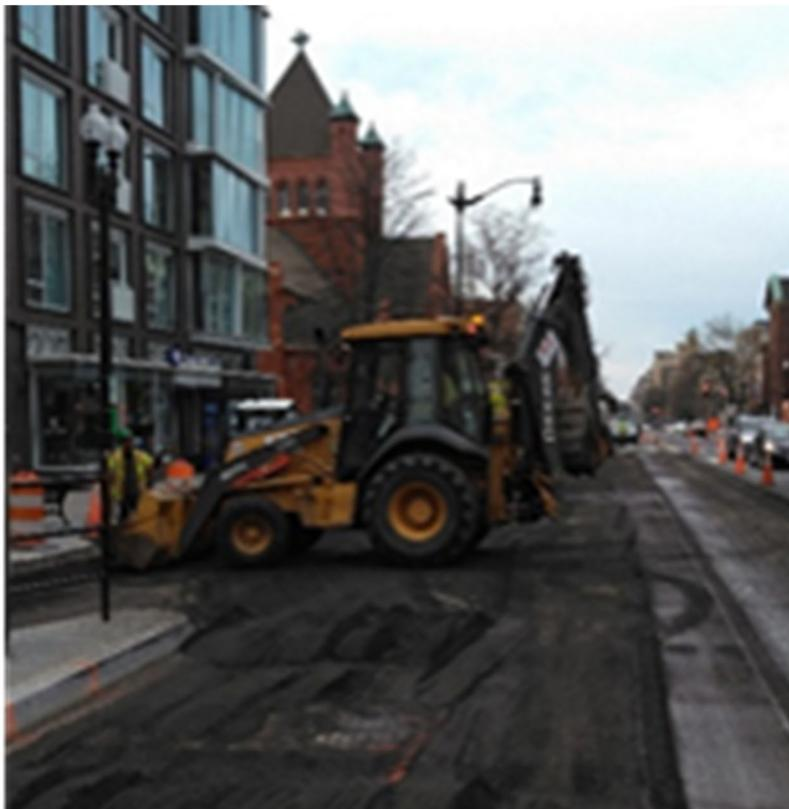
Manual pickup of milling spoils near Corcoran
