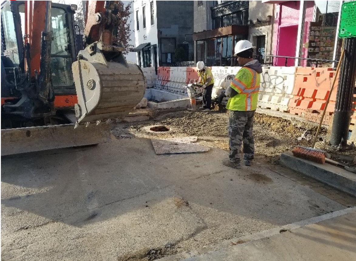
Omni backfilling and compacting sewer manhole M27
