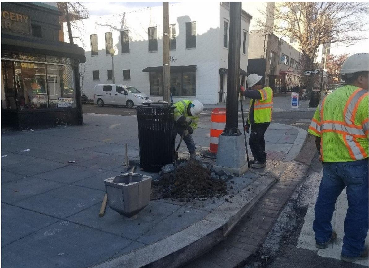
Excavation for SWC of 14<sup>th</sup> & Corcoran St flashing beacon foundation
