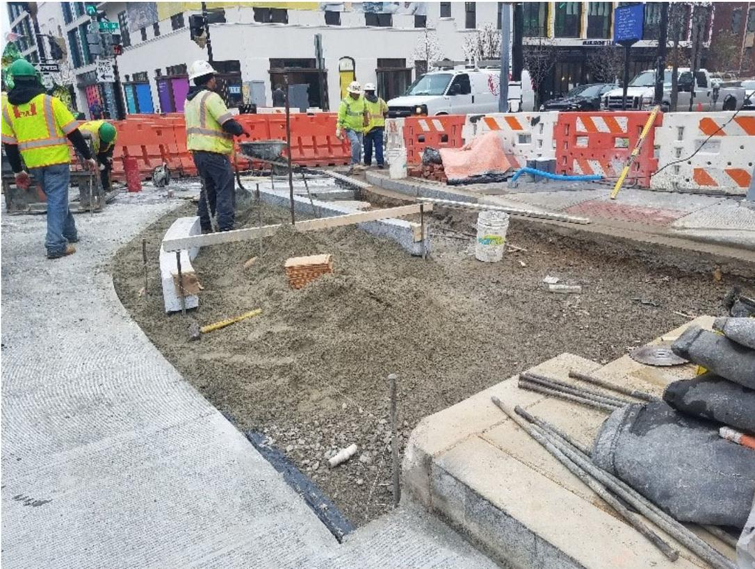
FMCC installing granite for bus island nose
