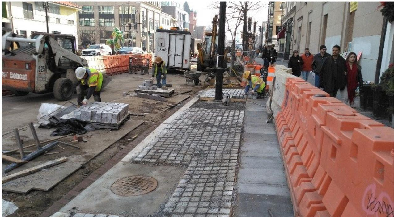
DEN installing Permeable Paver Sidewalk
