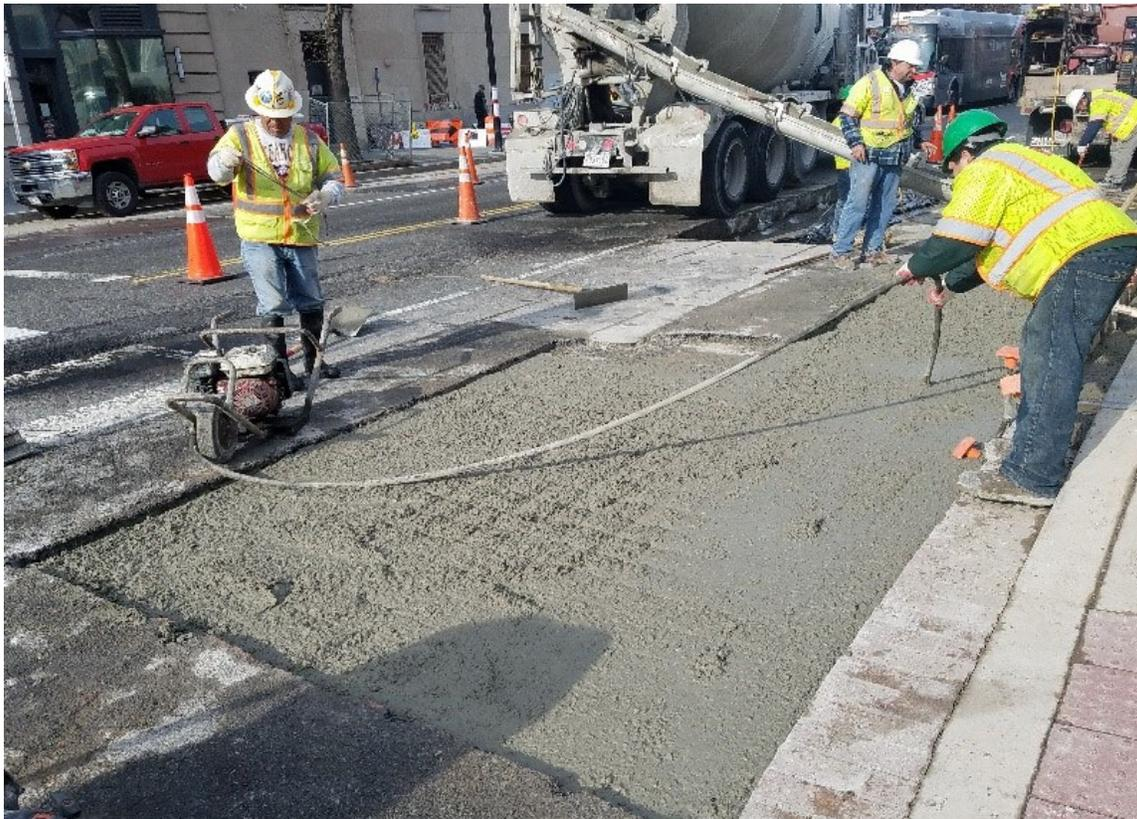
PCC Base concrete placement by FMCC
