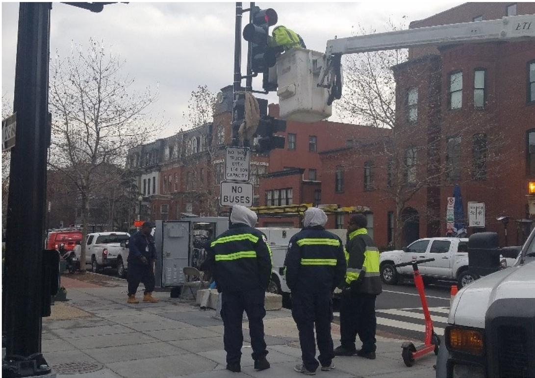
FMCC Electrical at Q St switching over to new signals with DDOT signal crew
