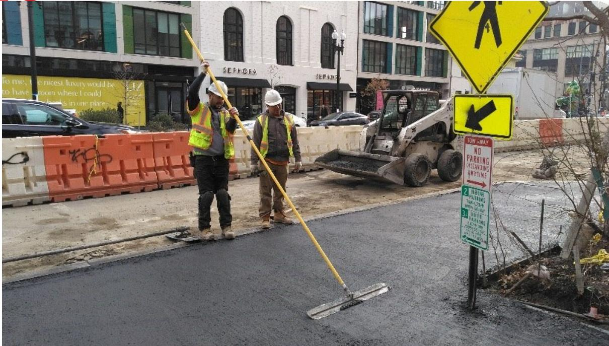
bull float on the proposed 4" PCC sidewalk between 1720 -1712 14<sup>th</sup> Street NW
