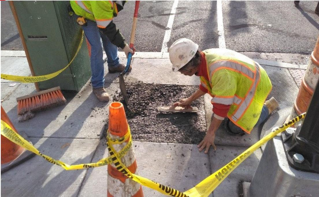
FMCC pouring 4" sidewalk at NE corner of S Street and 14<sup>th</sup> Street NW
