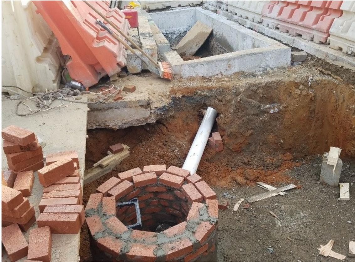
Bioretention planter #2 connected to MH27
