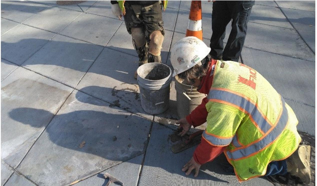
FMCC point and patching the temporary power cable conduit holes in the sidewalk at the NE corner of Rhode Island Ave and 14<sup>th</sup> Street NW
