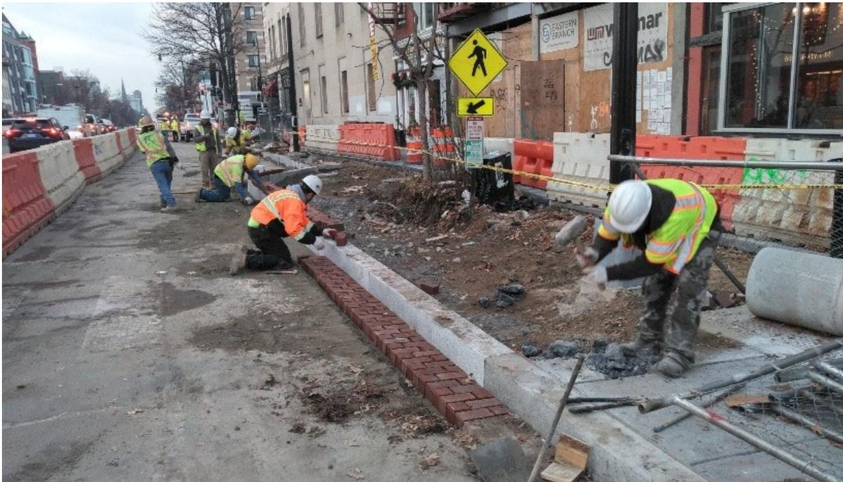
DEN installing the Brick Gutter between 1720 – 1712 14<sup>th</sup> Street NW
