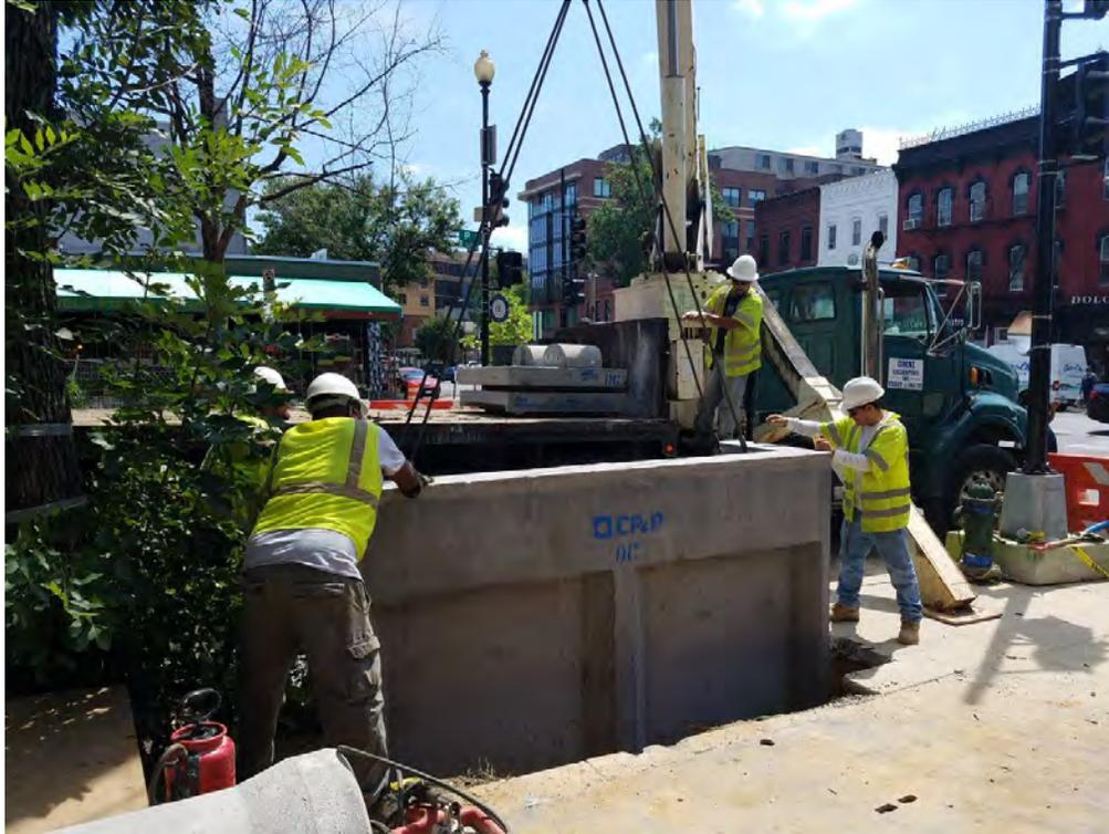
*Installation of Double Catch Basin t NE corner of 14<sup>th</sup> and P Street*
