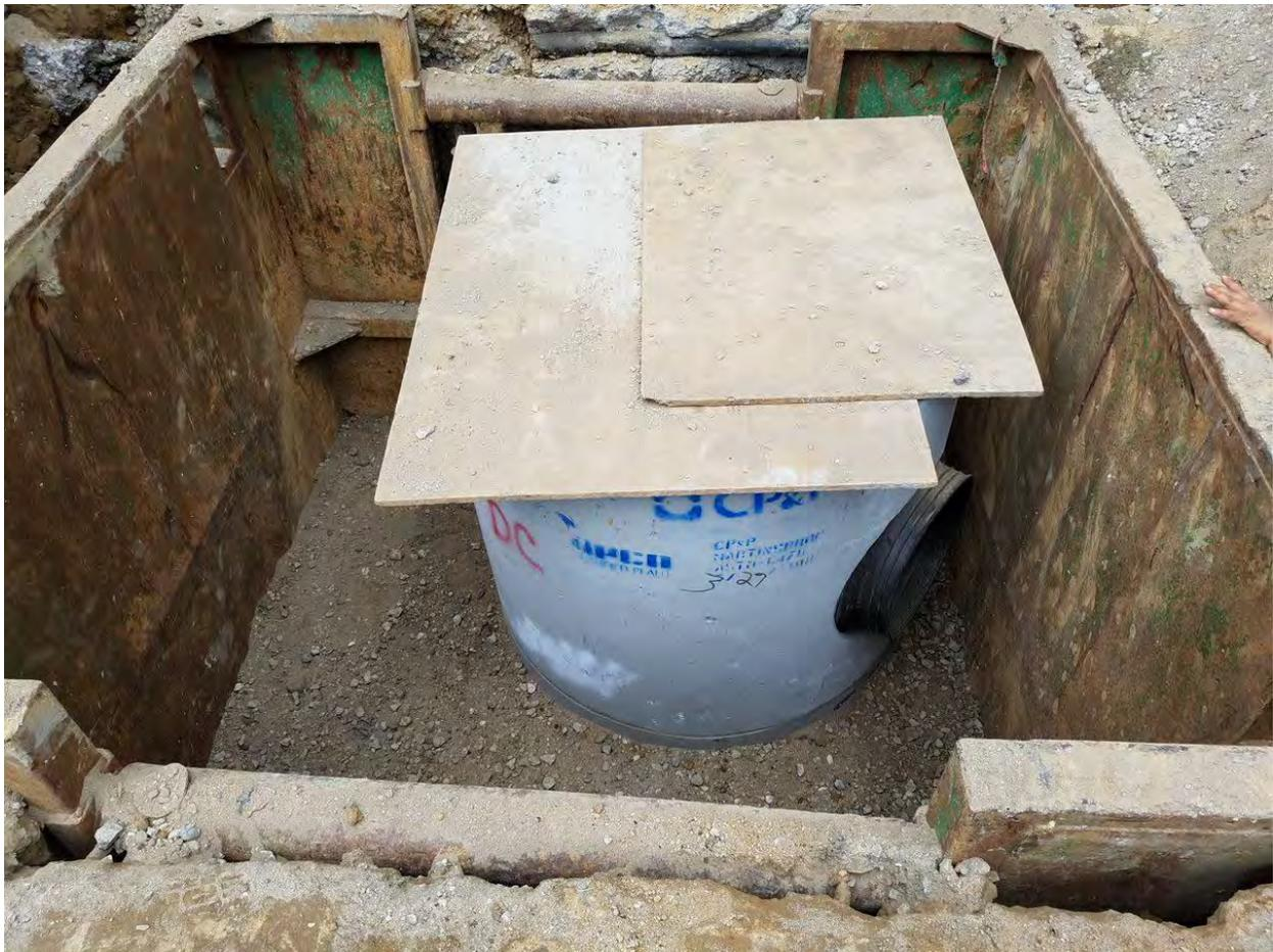
*Pre-Cast Structure for Combine Sewer Manhole MH-07 between P Street and Q Street Eastside*
