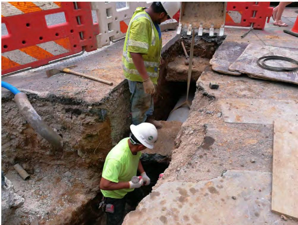
*Installation of 15" PCC Connection Pipe for the Double Catch Basin on the NE Corner of P Street*
