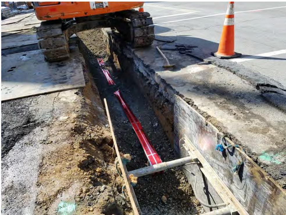
*Placing Metal Tracking Tape in between backfill per Specifications*
